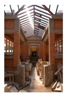
All told, King Bros. Masonry used 130 3,000-pound "super sacks" of QUIKRETE<sup>®</sup> Type N Mortar, formulated with white cement, Type S hydrated lime and aggregate from Frey Sand & Gravel, in addition to 120 "super sacks" of QUIKRETE<sup>®</sup> Type N Mortar, formulated with white cement, Type S hydrated lime and buff-colored masonry sand.
