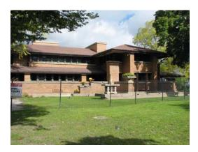
The project, the third in the four-stage restoration/rehabilitation plan, focused on rebuilding masonry walls, restoring face brick and matching mortar for the interior "backup" brick on the 10,000-square-foot main house, Martin House, and a 100-foot-long covered walkway (pergola) connecting the Martin House to an interior garden in the complex's glass-roofed conservatory.
